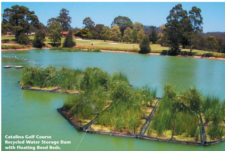
reduction of nitrate to nitrogen gas. The microbial activity also assists in the removal of phosphorus and heavy metals from the water by aggregating these free floating elements, they then settle out of the water and eventually become part of a sludge layer on bottom of the pond.
