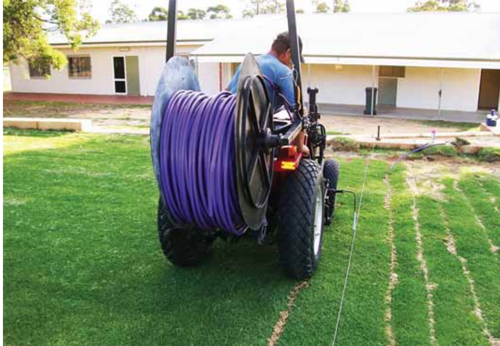
Installation of the subsurface irrigation system at Mundaring Shire Oval
