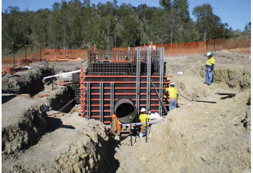
Work on the Caboonbah valve pit by Western Pipeline Alliance
